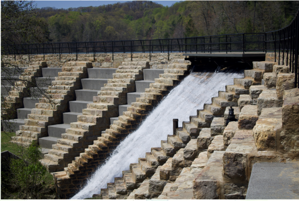
Bays Mountain Dam at Kingsport Reservoir
