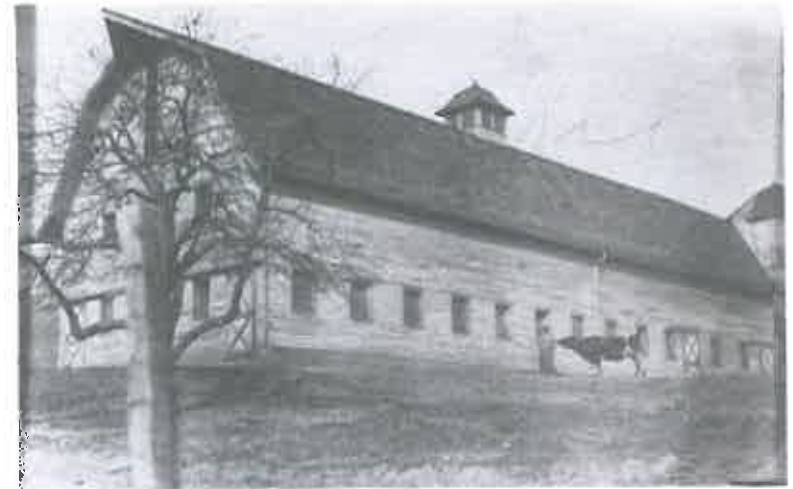
The large dairy barn of Wallace Farm. Secured in 1918, the 300 acre farm provided dairy products for the college and local community. The school was forced to sell the farm in 1938, however, in the depths of the Depression.
