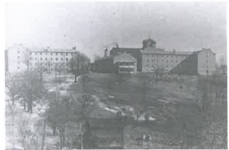
The Morristown campus in the 1920's, as seen looking east. This photograph shows the backside of New Crary Hall, Kenwood Refectory, and Wallace Hall. The tower of Laura Yard Hill Hall looms in the background.
