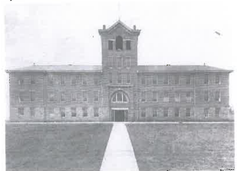
Laura Yard Hill Administrative Hall, named for Judson Hill's wife and completed in 1911 after ten years construction, was built with bricks made on campus. From its opening until the present, the building has served as the central campus structure, housing classrooms, main library, bookstore, auditorium, and administrative offices.
