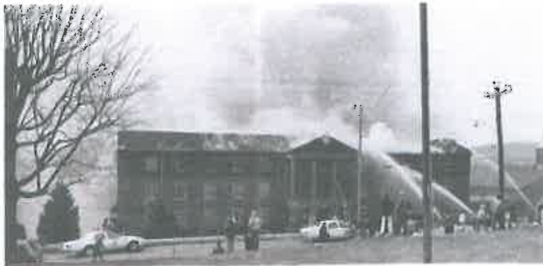
Fire struck the Morristown College campus once more in February, 1983, when Wallace Hall was set ablaze due to faulty wiring. The building has since been restored.
